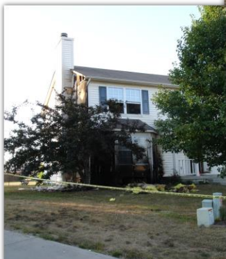
A/B corner from street
