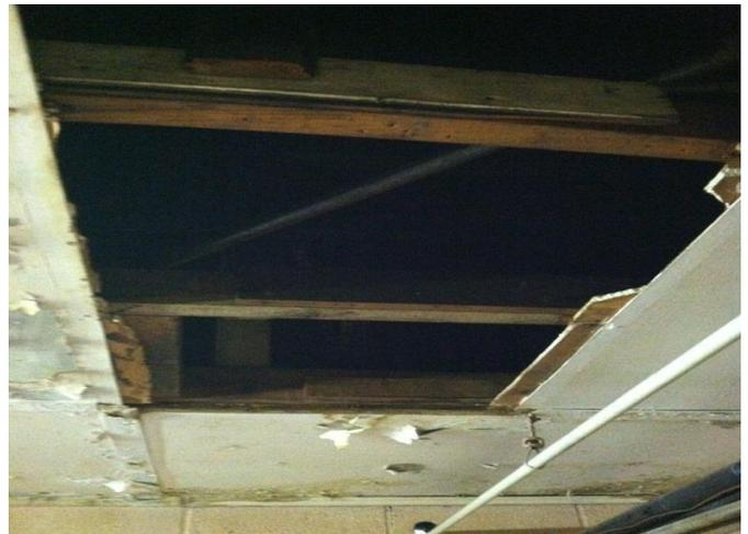
*Missing or damaged tiles on this basement ceiling will severely expose the first floor rafters in the event of a basement fire. (Photo by Author)*
