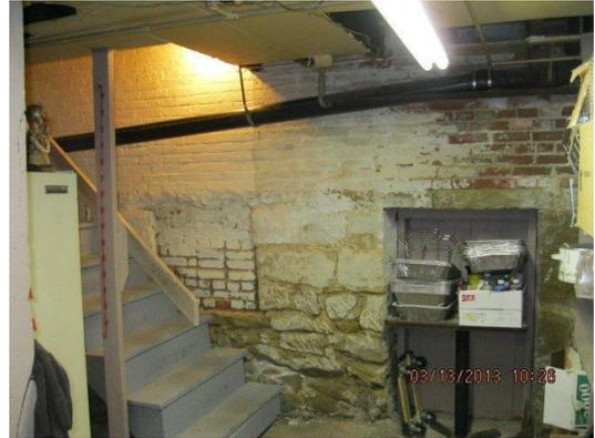
*Basements in continuous ordinary construction occupancies could be interconnected. This photo shows a flimsy piece of wood paneling covering an opening between two basements. (Photo by author)*
