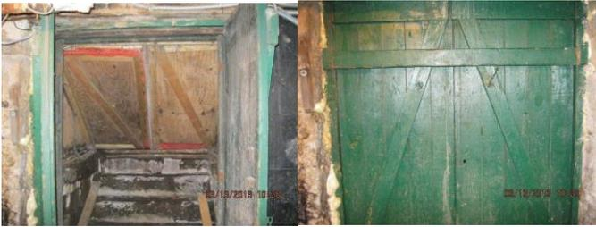
Basement forcible entry concerns: The photo on the left shows an interior shot of the exterior basement door, after you force these doors you are faced with another fortified door. These are two common security obstacles you may face; the key is to get into your buildings prior to the fire and see what you will face at 0200 when the fire call comes in.
