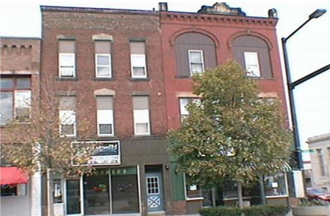
*A typical mixed-use ordinary construction building in author's response area, these two buildings were once separate now have interior walls on the second and third floors which house apartments have been removed making a single continuous structure above the still separate businesses on the first floor. (Photo by author)*
