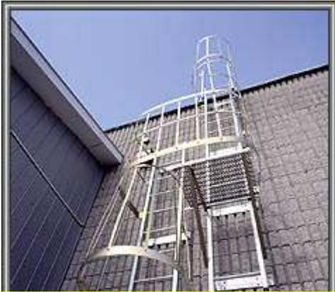
OSHA 29-CFR-1910.27 has a laundry list of requirements for FIXED LADDERS. Knowing where and how they are maintained in your first due, can help gain access to various areas. Having a basic understanding of fixed ladders can help you with perform a ladder size up and determine if this is an option.
