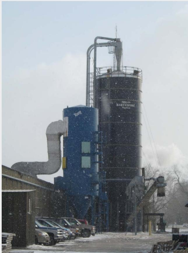
This Harvestore silo stores sawdust in a modified non-oxygen-limited fashion at a hardwood millworking facility. The sawdust is then conveyed from the silo to fuel a woodwaste-fired boiler.
