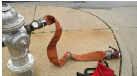
Next, begin to make the connection using the 3-inch discharge as you stand pipe. We utilize a short section of 3 inch to a gated wye and deploy 1 3/4 in our stand pipe racks. We also use an inline pressure gauge to know how much water we are getting on the line. If you are using 2 1/2 then your connection will be made without the gated wye obviously.
