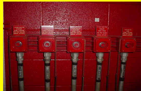
MANUAL DELUGE ACTUATION STATIONS
