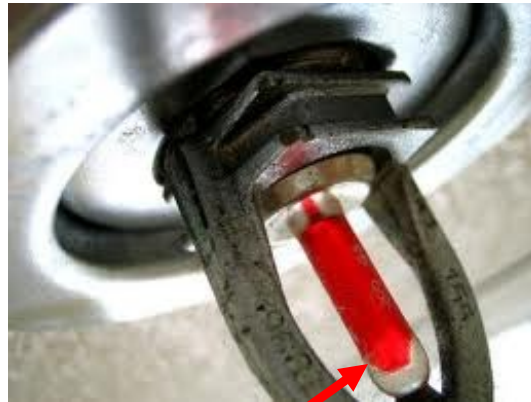
FRANGIBLE BULB SPRINKLER HEAD
